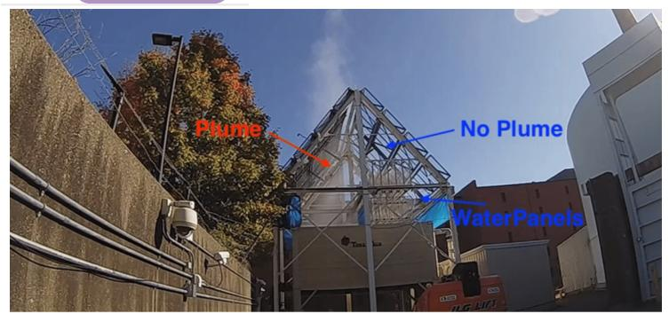
The cooling tower of MIT's nuclear plant was used to demonstrate the effectiveness of the water recovery system. The right side of the tower has the new system installed, completely eliminating its plume of vapour I Photo source Kripa Varanasi and Maher Damak
