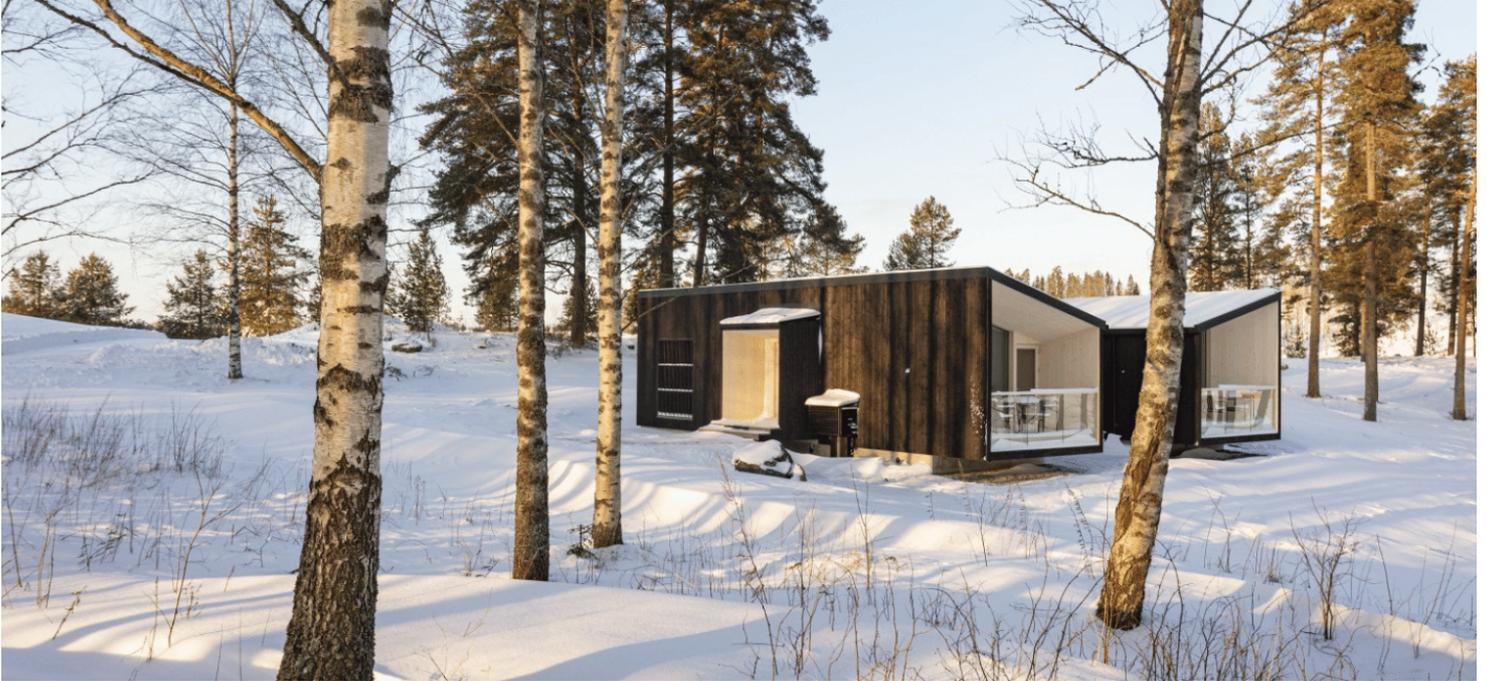
Each building was constructed using dark cross-laminated-timber cladding, which blends in with the natural environment | Photo source [Studio Puisto](#)
