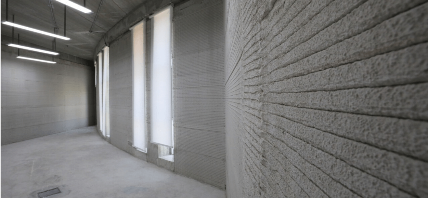
The 3D-printed building | Photo source Apis Cor
