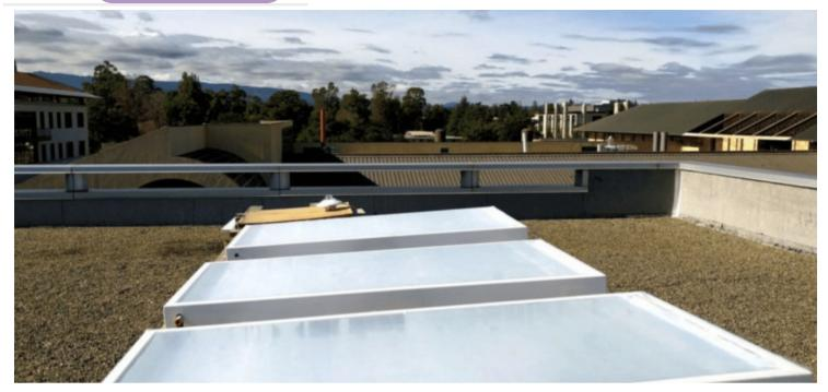
At Stanford University, SkyCool's co-founders Shanhui Fan, Eli Goldstein and Aaswath Raman invented a film-like material that facilitates the radiative cooling process. | Photo source Aaswath Raman
