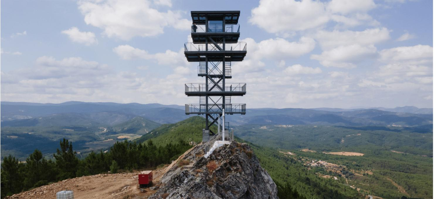
The tower is made from a lightweight steel structure that is divided into platforms at various heights | Photo source [Daniel Sousa](#)
