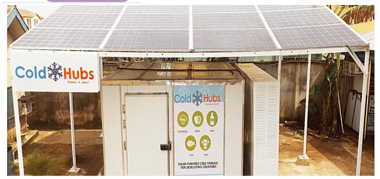
The design employs rooftop solar panels that can generate enough electricity to power the units in all weather conditions | Photo source Cold Hubs
