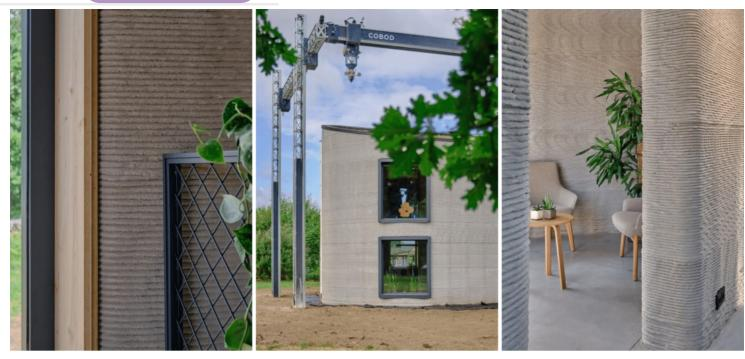
The prototype building was constructed in one piece using a huge gantry printer | Photo source © Kamp C & Jasmien Smets
